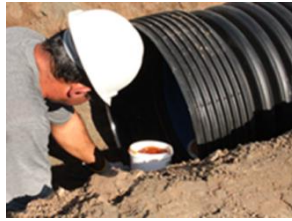
Figure 38 - Application of lubricating paste
