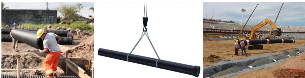
Figure 45 - Unloading and handling by hand and with nylon straps
